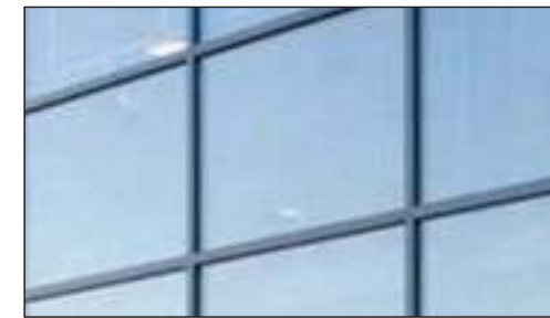
Curtain Wall Grey Mullions
