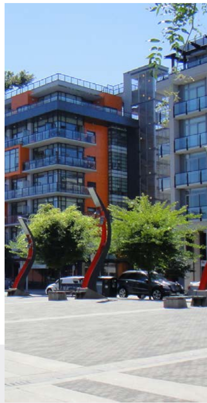
High-Quality Building Design
